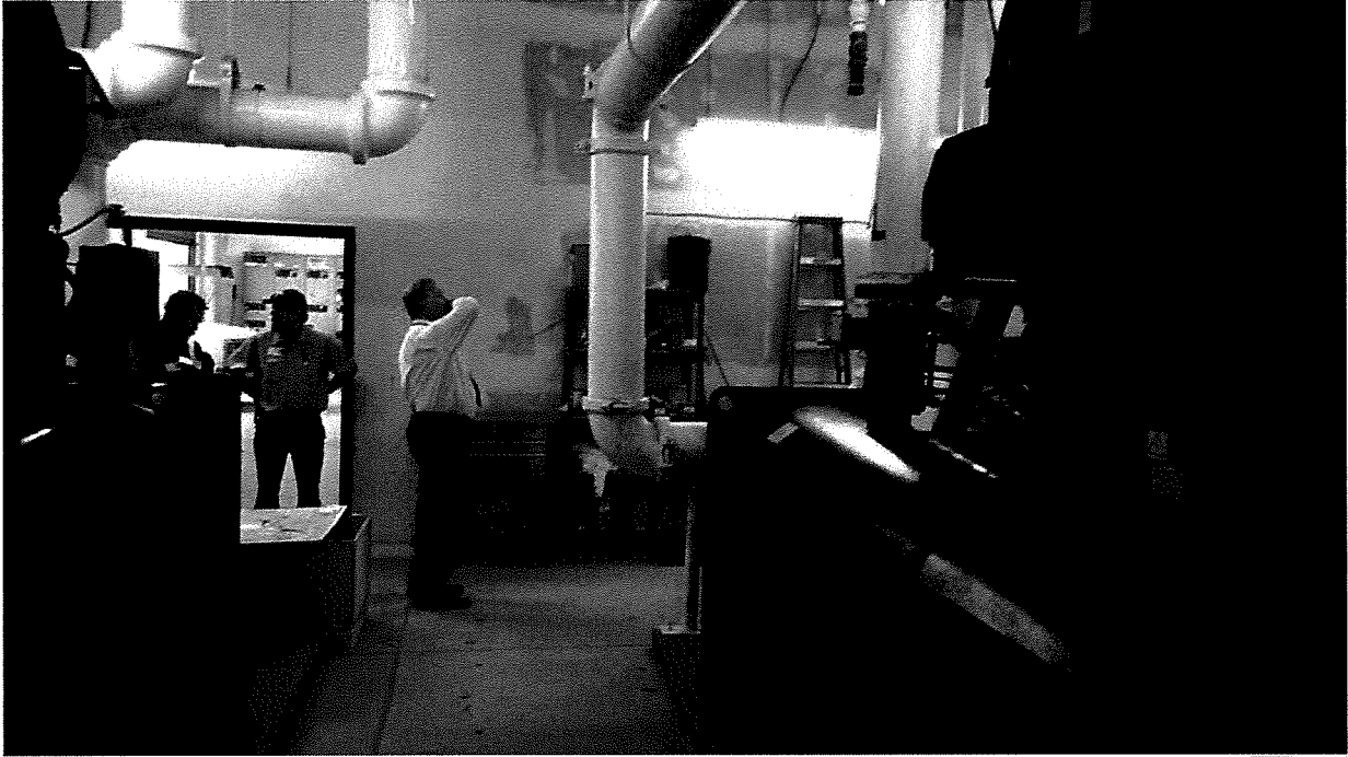
Photo 2: Existing CH-1 on right, CH-2 to left. Note lack of opening to move CH-1 in/out of the mechanical room. The wall behind the photographer in this photo is masonry.
